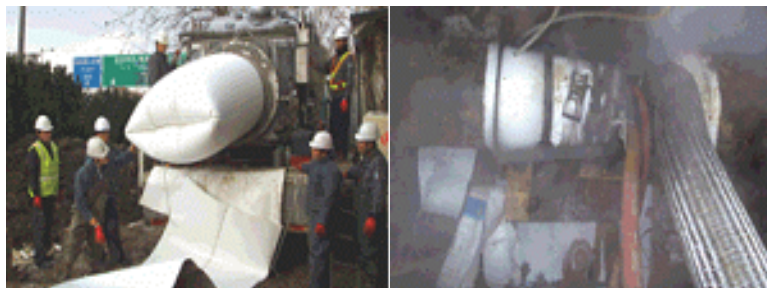
Fig. 5. Tube Inversion and Steam Curing Process of Conventional CIPP.
